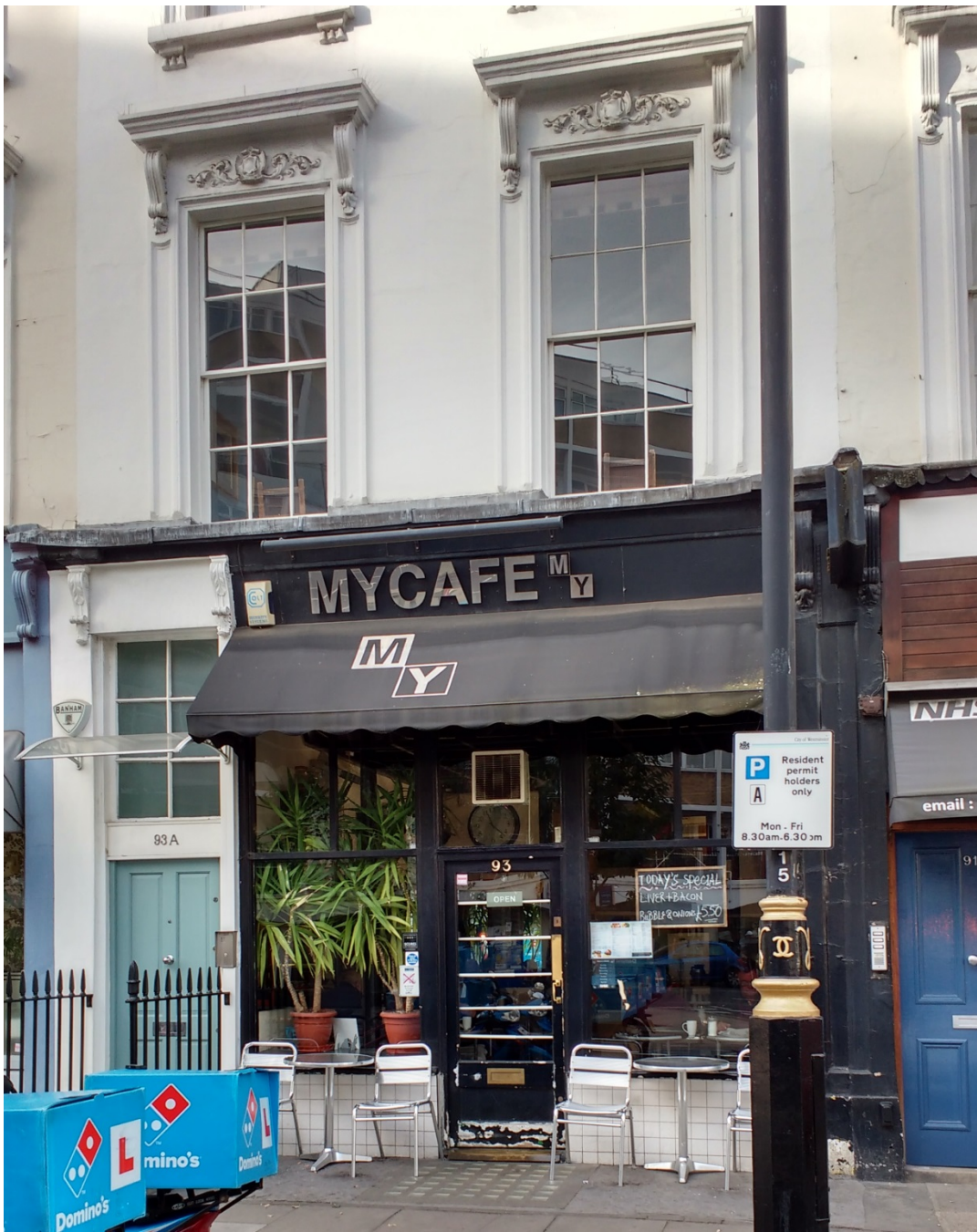
No. 93 Charlwood Street
